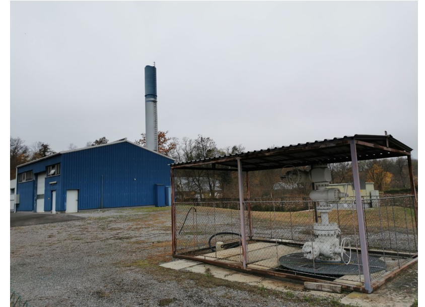
Former geothermal DH system Fuerstenfeld, Austria (photo: Gregor Goetzl)
